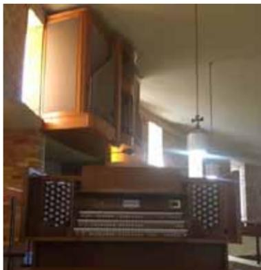
The installation was complicated, as the console had to be lifted into a high gallery and the speakers were placed into a custom speaker cabinet mounted on the wall, complete with a pipe façade. The flexibility of a wall mounted cabinet in this oval shaped chapel gives us the ability to mix the direction of the speakers to blend the sound and create an ambience that makes the organ sing.
